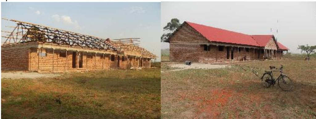
Phase 3 involved the completion of the concrete floors, the plastering, painting and fitting of the windows and doors.
