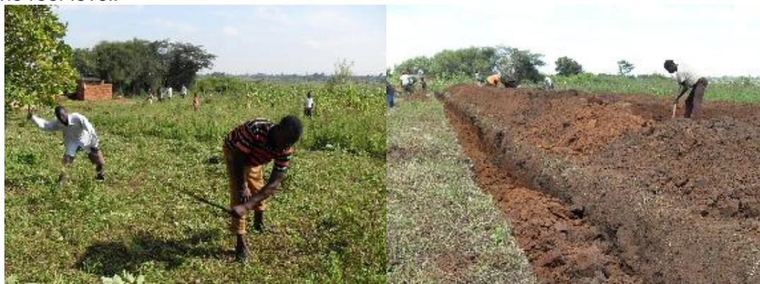
The foundations were dug down to the stones/ rock level to provide a strong base for the foundations which were set with concrete.
