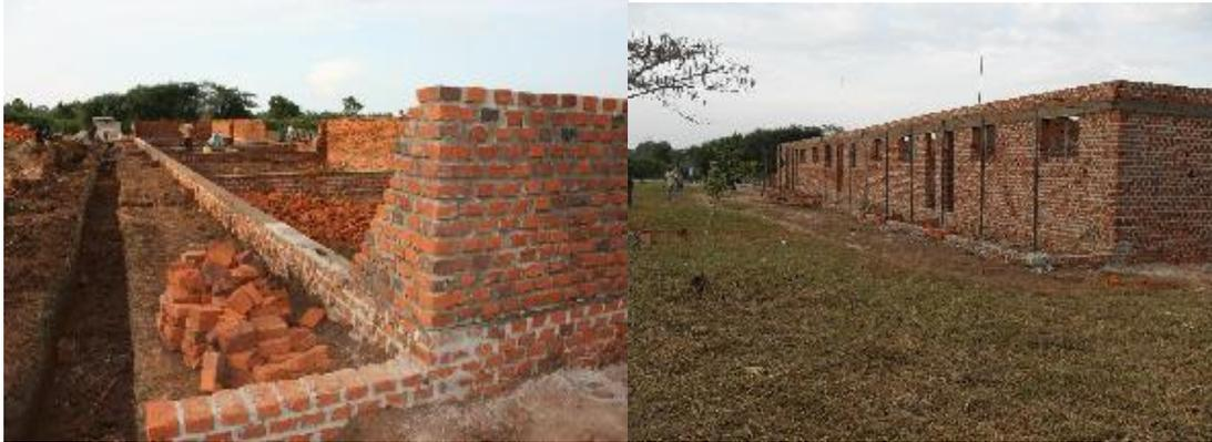
After the walls had time to set and strengthen, we began the process of making the concrete beams for above the windows. The external poles and foundations for the veranda were also set and provided the support for the roofing in phase two.
